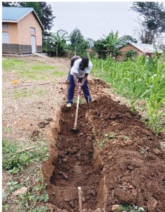
Digging trenches to retain water and avoid erosion
